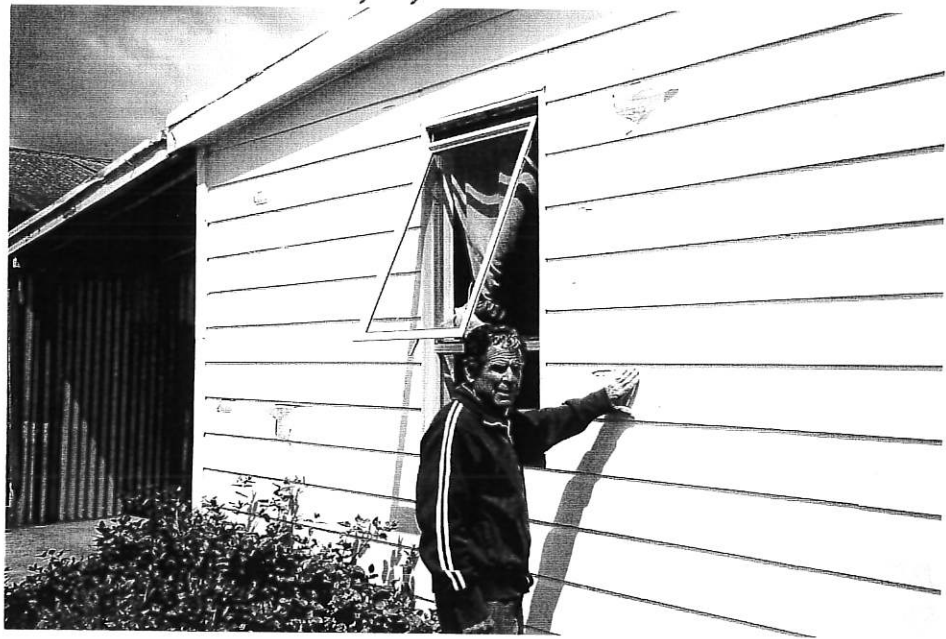
Paint on the east side of the house is flaking off. (No undercoat on the primer)
