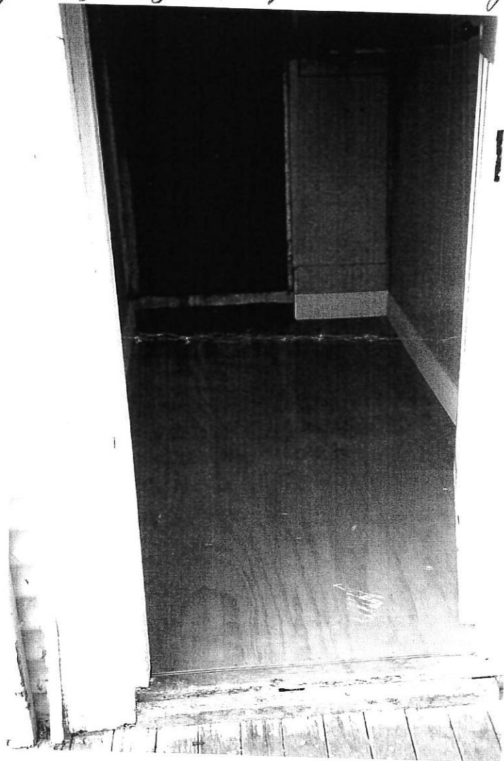
New floor replaces the rotten one in the shearer's quarters
