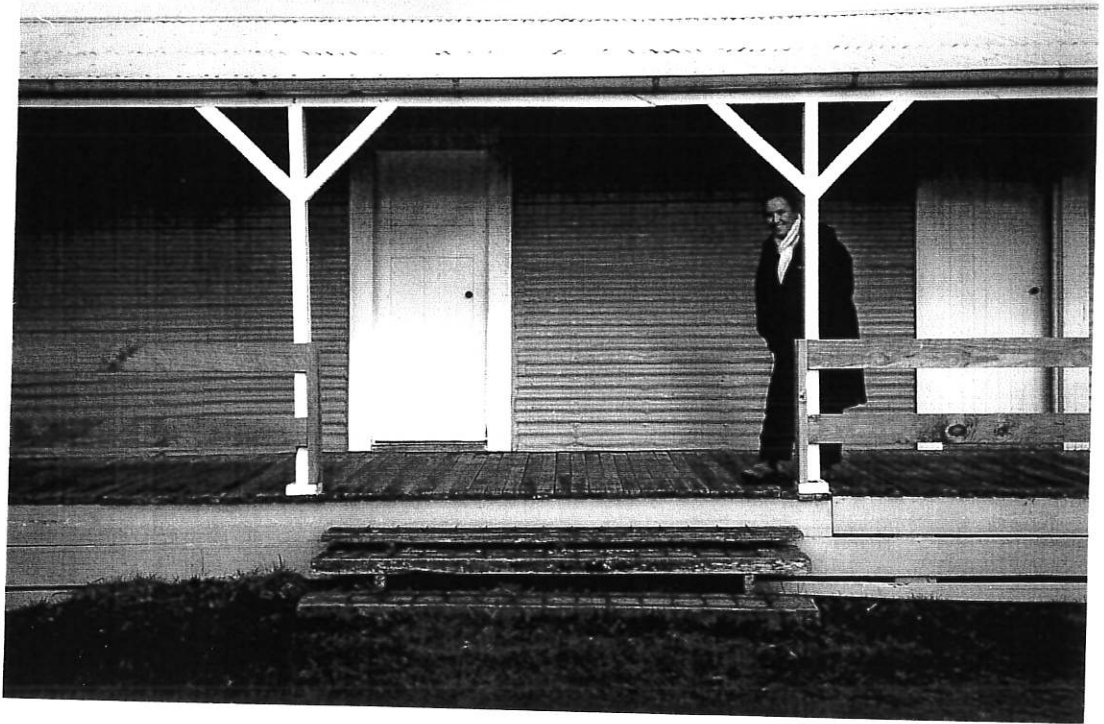
Rose Wharehanga inspecting the repaired verandah floor at the shearer's quarters.
