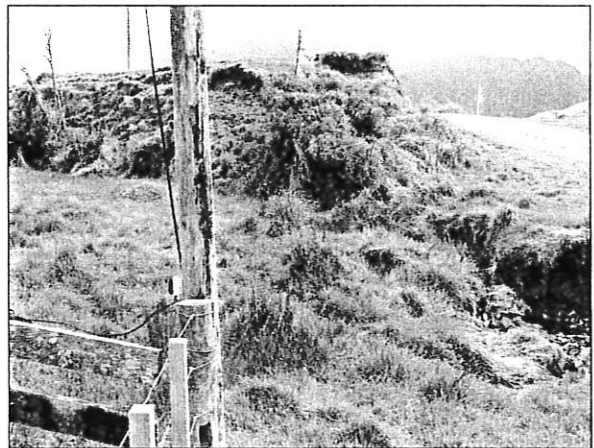
Road fence which is not in place
